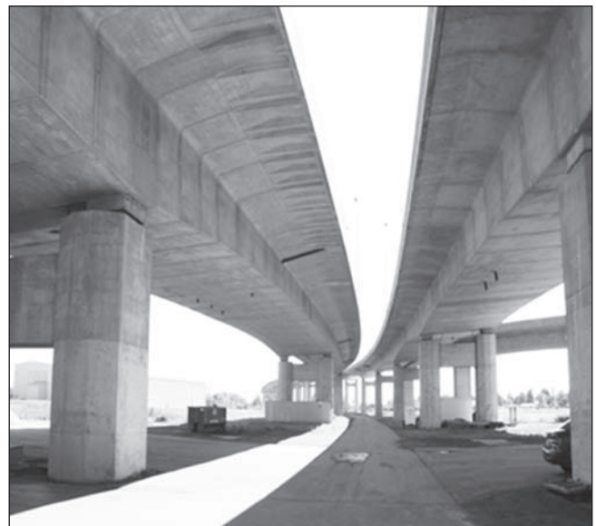
Figure 1. Typical PSC box girder bridge
