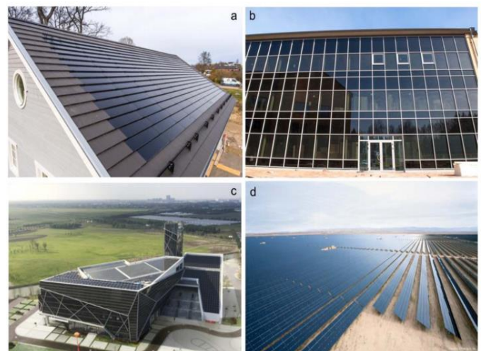
Fig -1: (a) Residence with CdTe PV tile in Europe; (b) office building with semi-transparent CdTe panels in Europe; (c) exhibition hall with 5556 m 2 of standard, semi-transparent, and artistic CdTe panels in Asia; (d)
