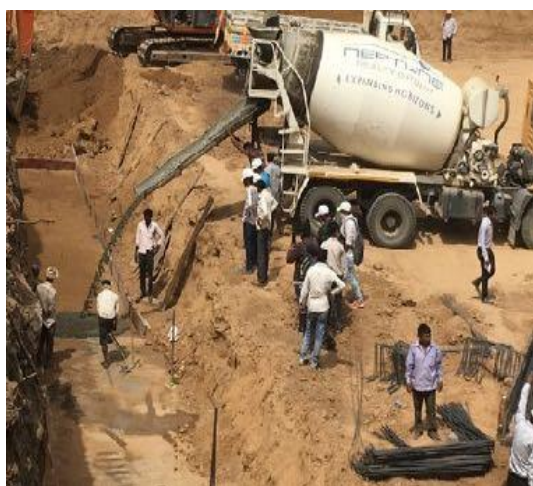
Picture 4.37 Students monitoring the concrete pouring project practicum.
