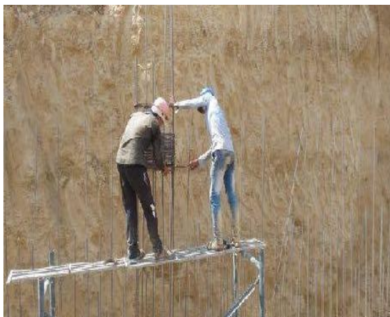
Picture 4.32 Students discussing and monitoring RCC Foundations Construction
