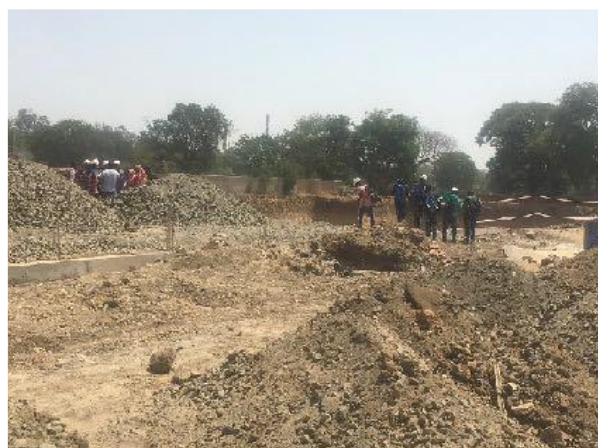
Picture 4.18 Students interacting in a group as team members and monitoring excavation field practicum under the supervision of site supervisors.
