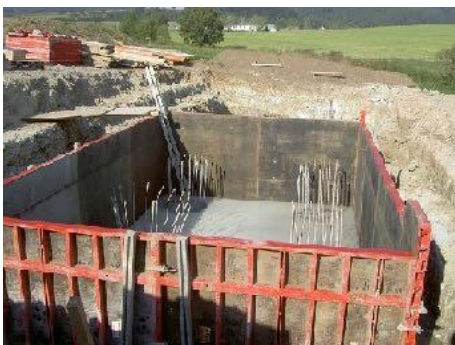
Picture 4.24 Formwork for buildings Source: the constructor.org.
