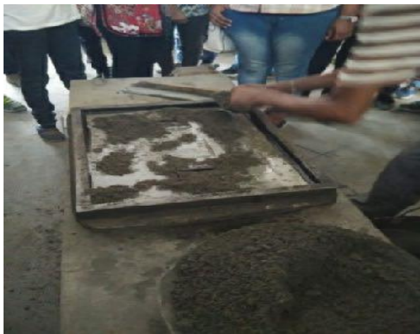
Picture 4.43 Students working on the pre casting mold for a precast unit at the Precast manufacturing plant for assigned project practicums
