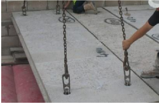
Picture 4.42 Precast Concrete Floors. Source: Wikipedia.com
