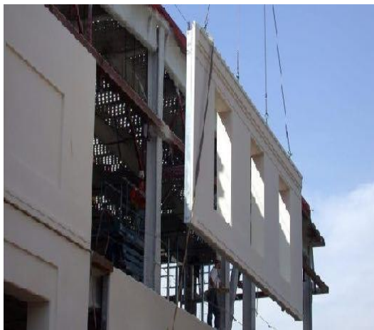
Picture 4.41-b Precast Concrete Wall Construction Source: Wikipedia.com
